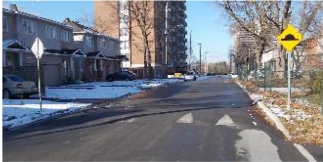
Figure 2 - Speed hump and signage
