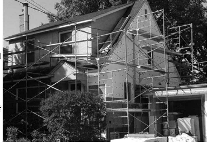
The house had a polka-dot look when the insulation was nailed in place. Later, it was covered in a smooth stucco.
